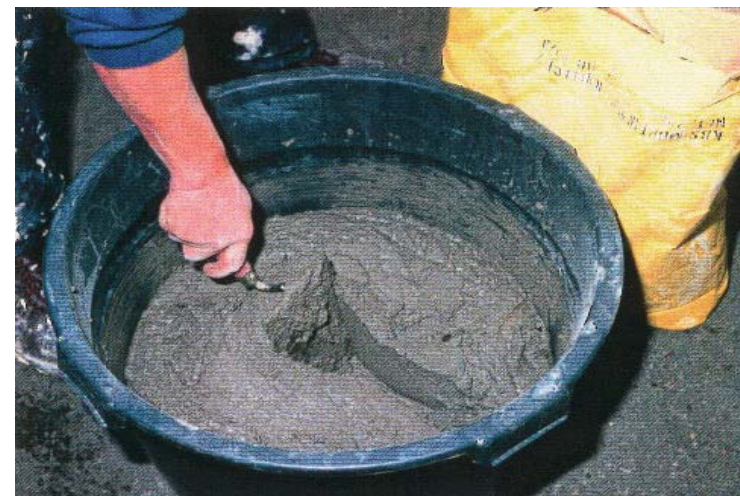
Mixing KBS Mortar to the required consistency
