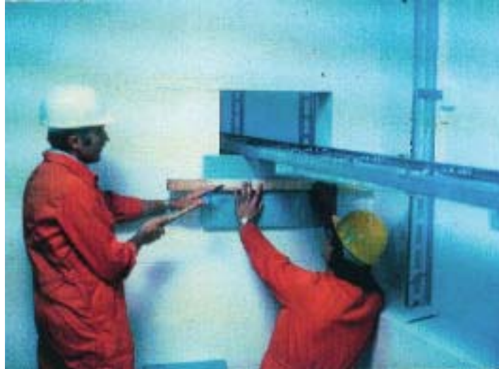
Attaching formwork to one side with hooks or nails
