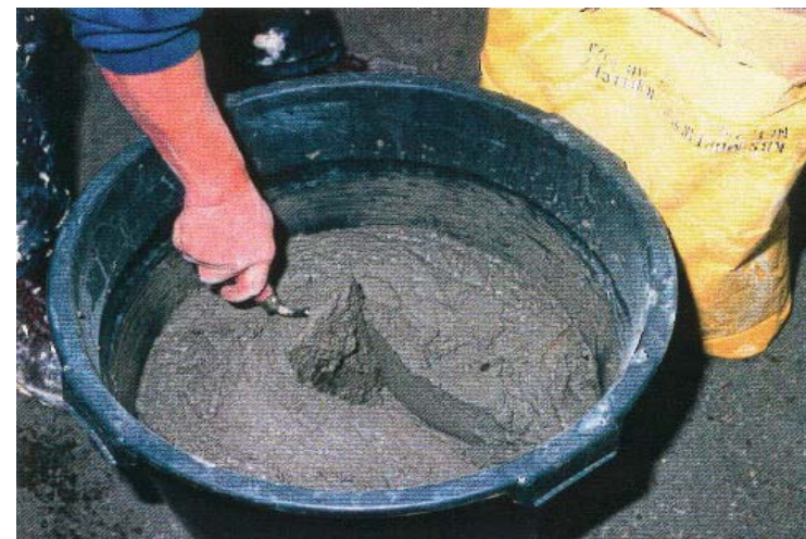
Mixing KBS Mortar to the required consistency
