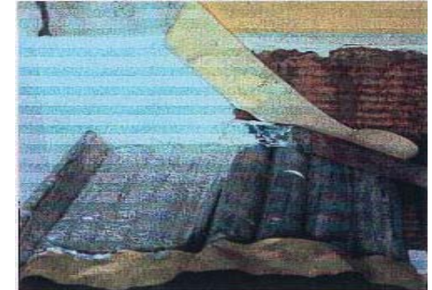
Spray the panel with KBS Cable Coating. Remove masking tape. Check to ensure all cables are coated on all sides.
