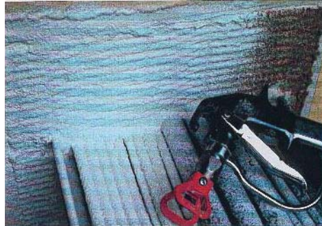
Spray the panel with KBS Cable Coating. Remove masking tape. Check to ensure all cables are coated on all sides.
