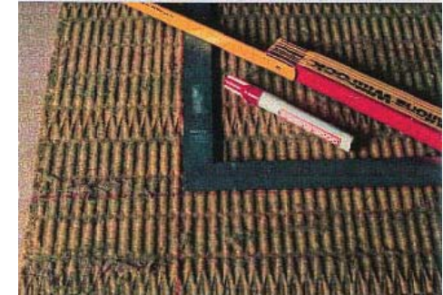
Measure uncoated panel and cut to size
