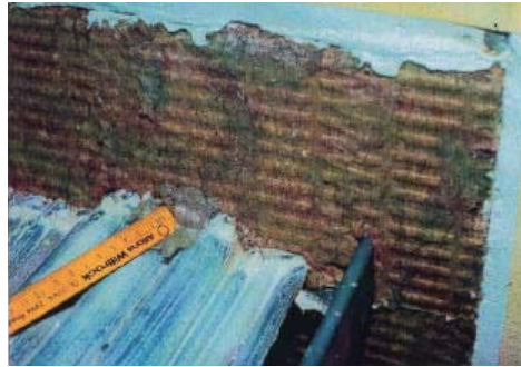
Seal small gaps with KBS Sealant before complete final coat.
