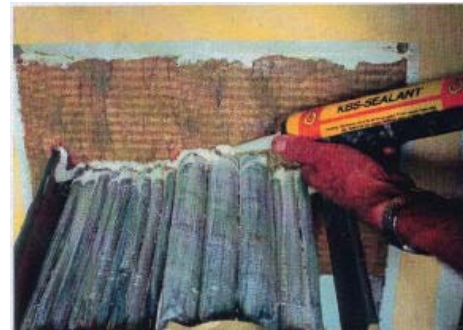
Seal small gaps with KBS Sealant before complete final coat.
