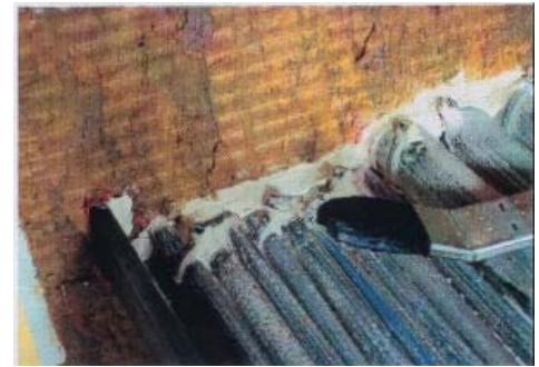
Use a wet brush to smooth the surface.
