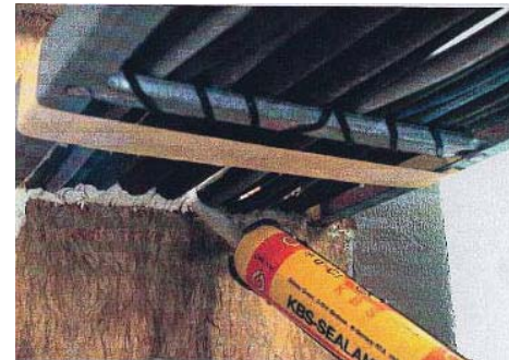
Working from the reverse side of the panel close all gaps with mineral wool and coat with KBS Cable Coating
