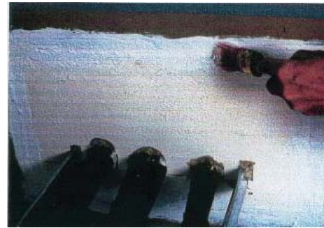
Coating the areas around the panel
