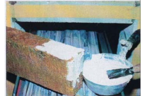
Apply KBS Cable Coating generously to Mineral Wool panels and to inside of opening.
