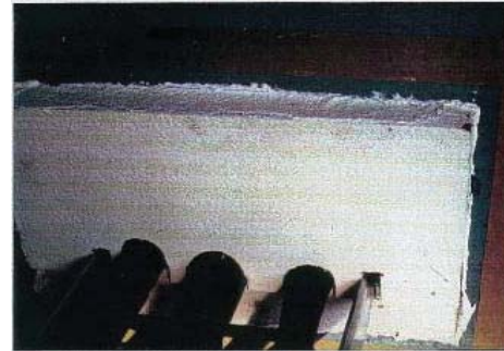
Moving panel into place
