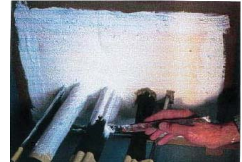
Coating the cables to complete the seal
