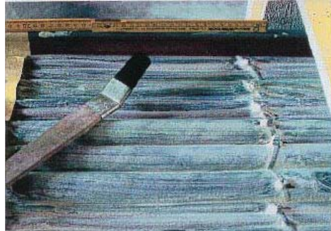
Apply a thin coat of KBS Cable Coating - brush or spray.
