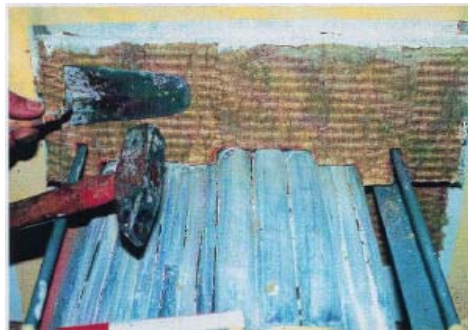
Push panel section into place - with a trowel or hammer.
