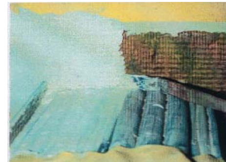
Spray or brush the panel with KBS Cable Coating. Remove masking tape. Check to ensure all cables are coated on all sides.
