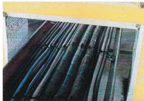
Using 30mm masking tape protect wall and floor openings.
