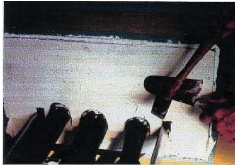
Placing pre-coated panel
