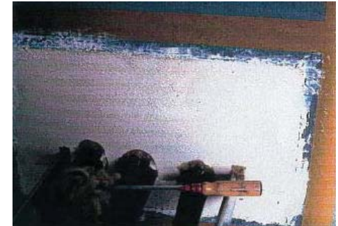
Making sure all areas are taped and ready for coating
