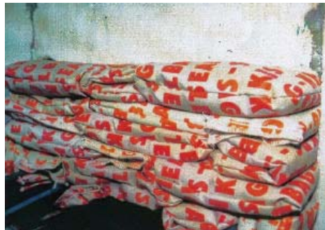
Completed penetration using KBS Sealbags
