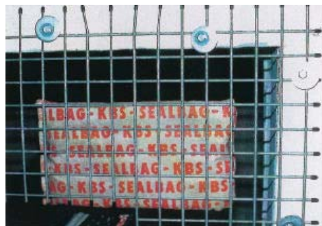
KBS Sealbags over a wire mesh base
