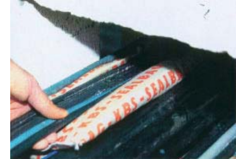
Placing Sealbags over and under the cables
