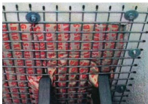
Completed KBS Sealbag floor penetration
