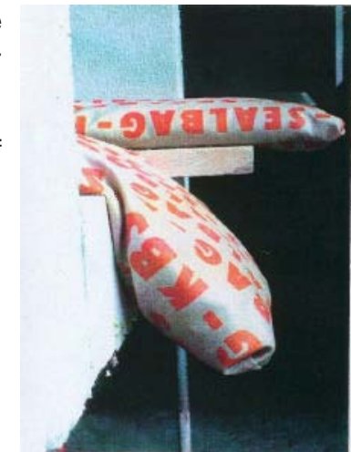
Extra support for wall under 240mm
