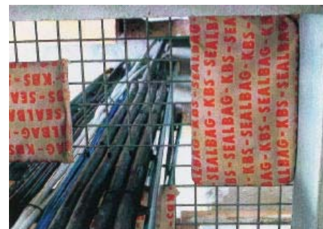
Open penetration with KBS Sealbags being placed.
