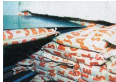
Finishing the application with steel plates
