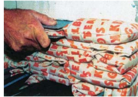
The use of 2 steel plates to finish off sealing the penetration
